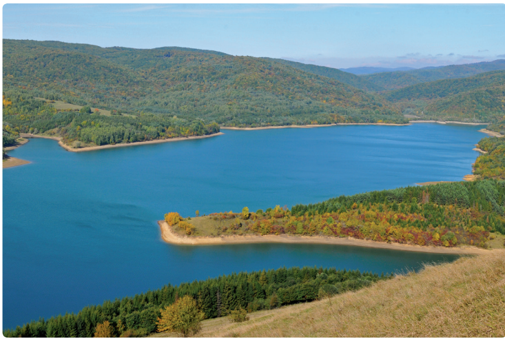
Starina Water Reservoir (C.Č.)
