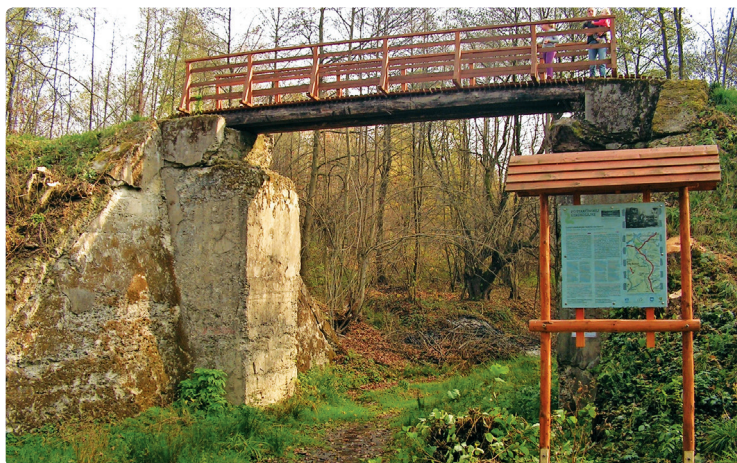
Barankowy bridge – Stakčín (M.B.)
